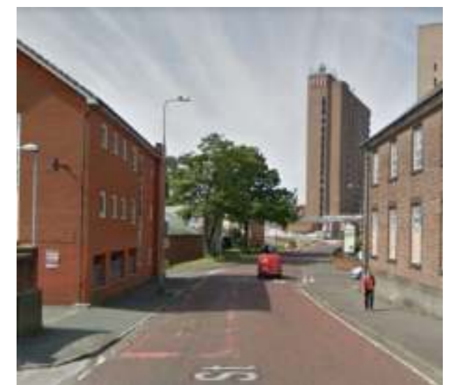
View towards Preston Bus Station from Percy Street.
