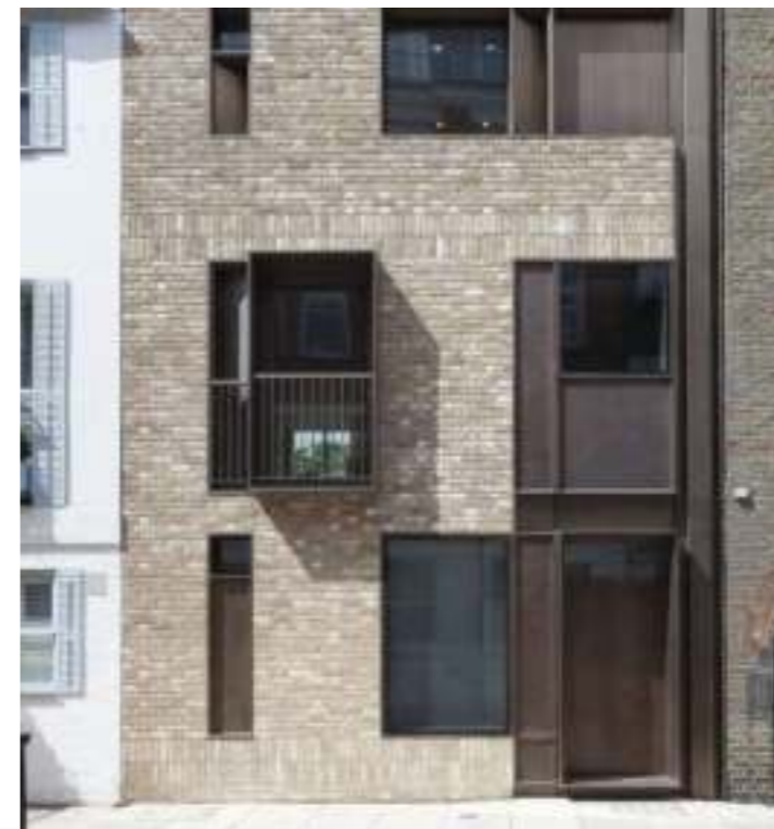
Buildings 2-3 storey (around Arkwright House)
