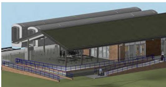
Access Preston. New railway station.
